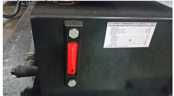
2.) Step 2. Check hydraulic level
